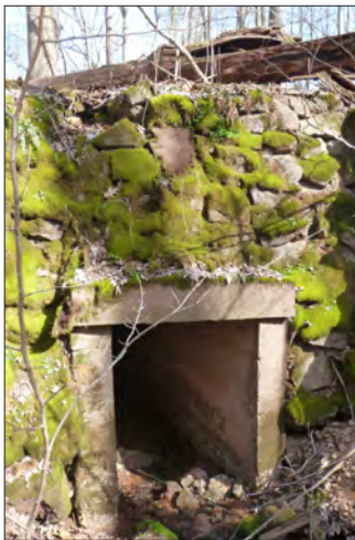
Keystone culvert built in 1923
