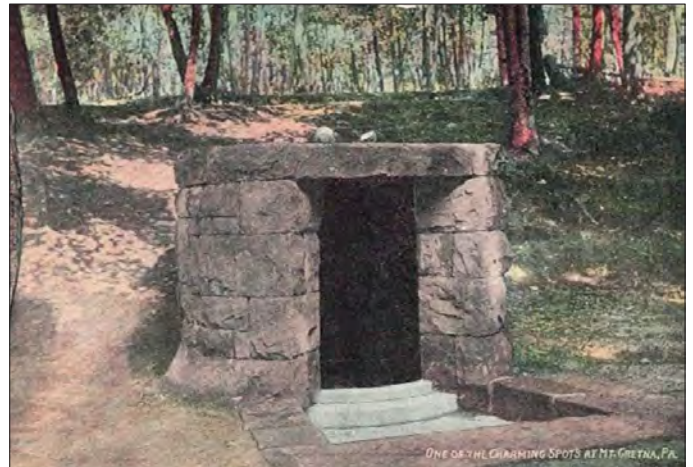
In 1884, Robert Coleman directed masons to enclose springs like the one pictured above, likely in the Mount Gretna Park, according to Jack Bitner’s Mt. Gretna: A Coleman Legacy. Photo from MGAHS Archives.
